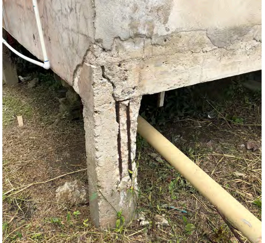
Foundation failure, house in Yabucoa.
